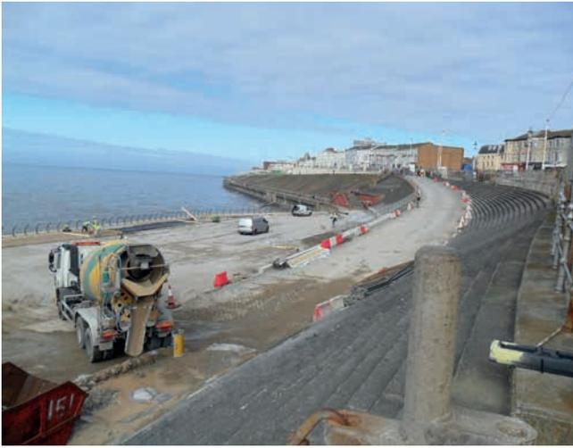
**4,000m<sup>3</sup> of Leca LWA** was used to fill the void between the existing sea defences and a new sea defence wall
