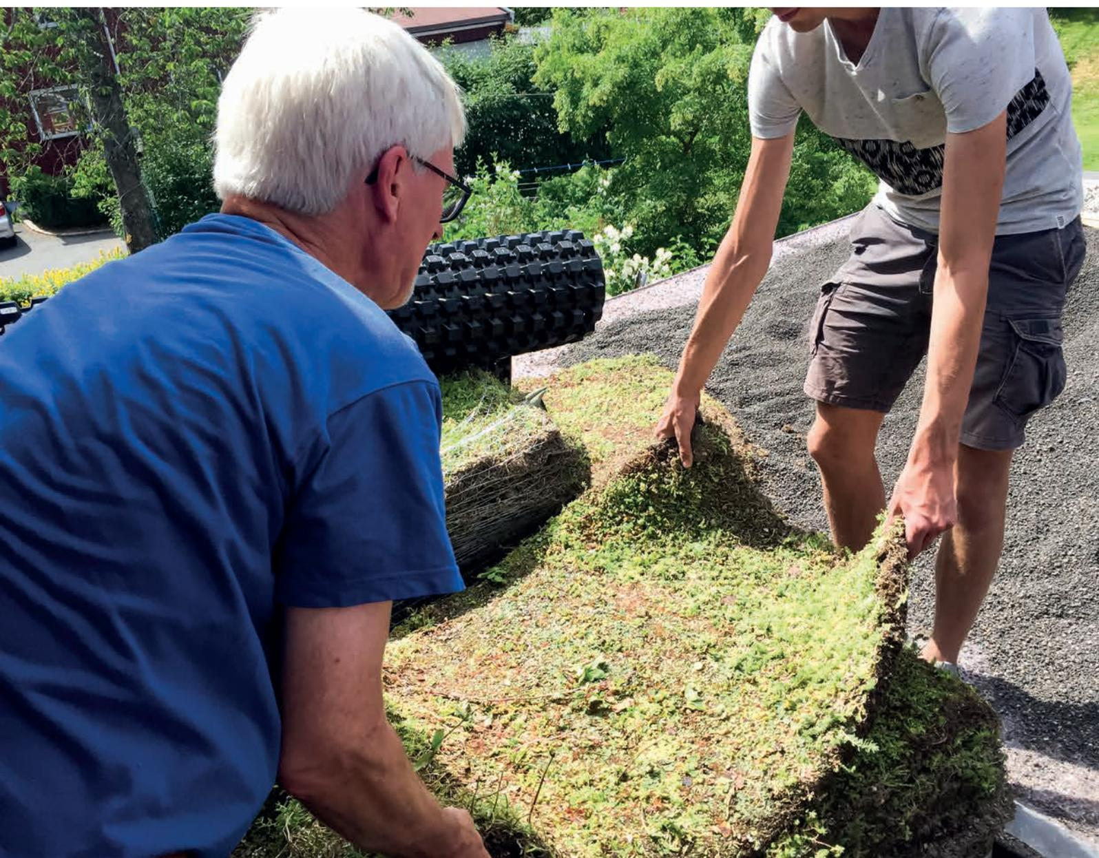
**Crushed Leca 0-6 mm** was used to maximize water detention when Bent C. Braskerud installed a green roof on his home in Oslo
