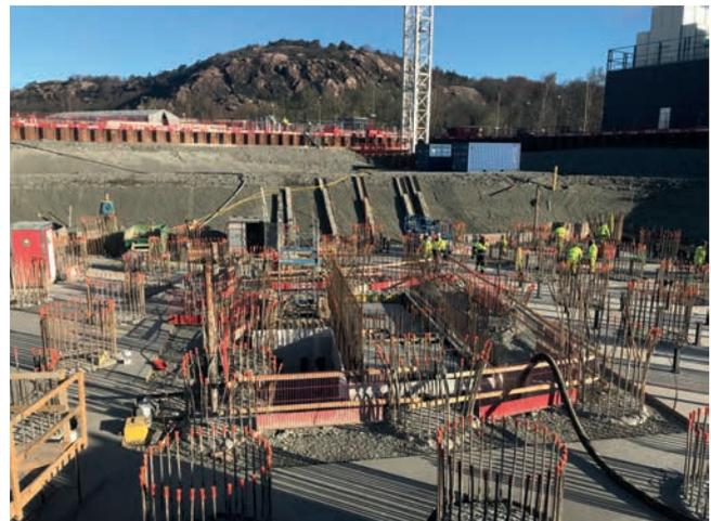
**Leca LWA being** delivered by blowing truck to the center of the tower foundation
