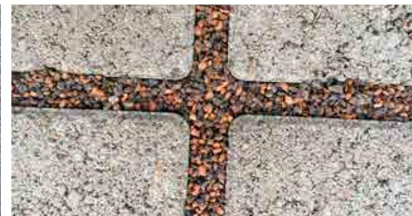
**The chosen Leca LWA** was crushed and extra fine to maximize the effect of the water absorption in the material.
