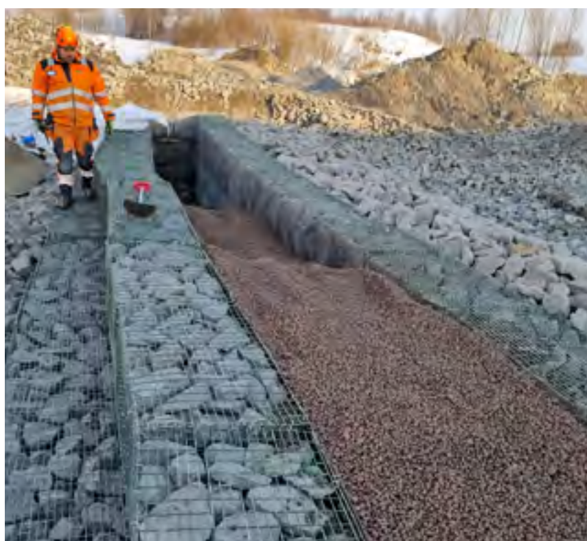
Leca LWA placed in the dam core, easy to replace.
