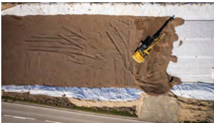
Leca LWA was compacted with a crawler excavator.
