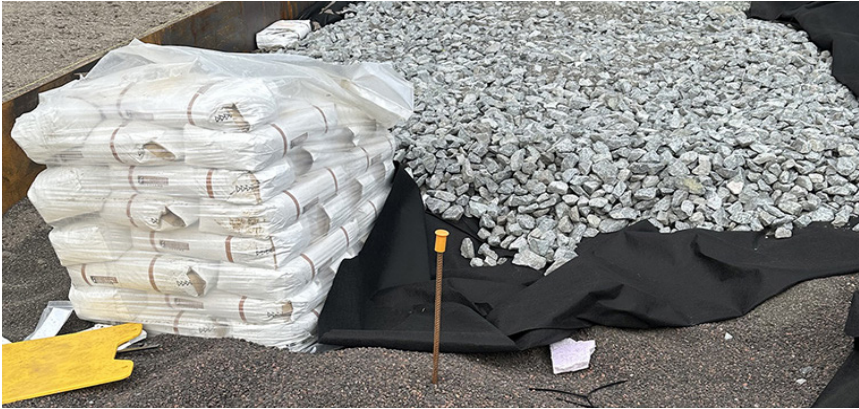
Above the concrete surface, there are green areas laid out with Leca® LWA 2/10, which is crushed for storage, drainage, and infiltration of stormwater.
