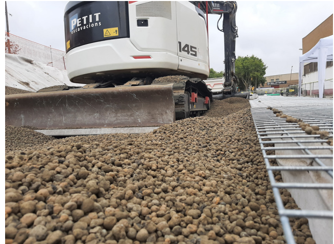
Compaction of the material using doozers
