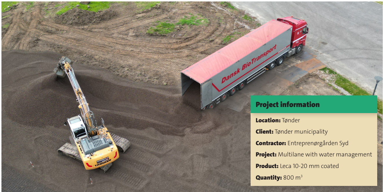
Delivered with a walking floor, each load can contain 93 m 3
