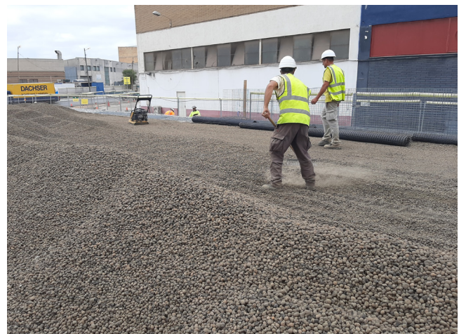
Manual spreading in areas close to walls
