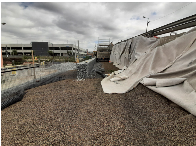
Arlita® containment through gabion walls and use of geogrids
