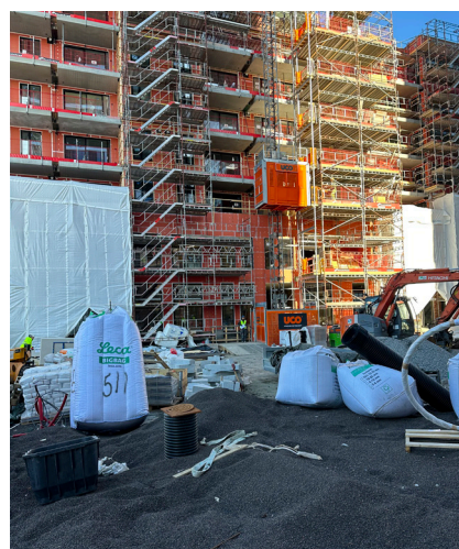
Leca® LWA contributes to the efficient drainage of water away from the building mass.
